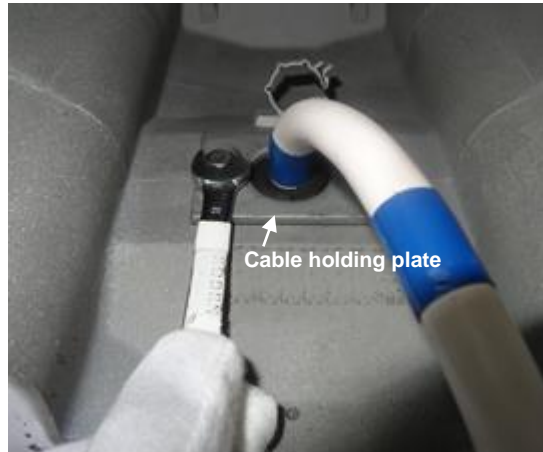
10) Attach cable holding plate and fix it with two bolts. (Tool: Wrench 8mm)
