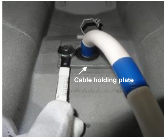
10) Attach cable holding plate and fix it with two bolts. (Tool: Wrench 8mm)
